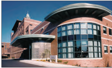
Photos above courtesy of DMR Architects, Hasbrouck Heights, NJ.
